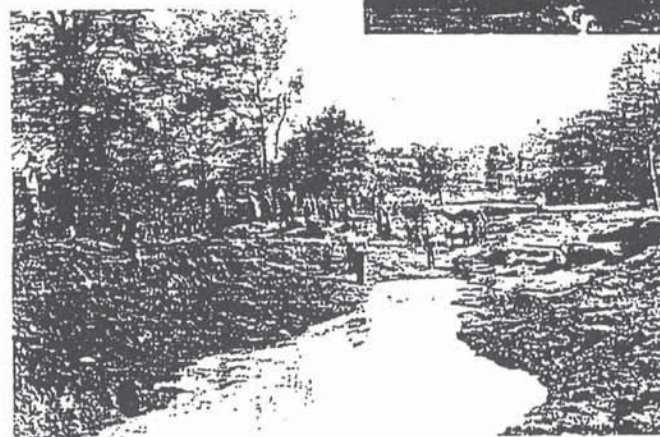
Immediately after explosion, water is entering new channel, whose banks will be smoothed and "stream-lined" by the speedier flow of water.
